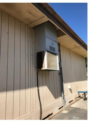
Photo 1- ADA hazard on a portable structure.
