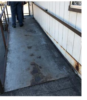
Photo 3- Visible corrosion on a ramp leading to a portable structure.
