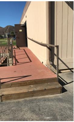
Photo 2- The building step is unsafe. Handrail is required
